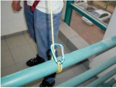
Make sure that the line is fixed properly by pulling hard on the line.
