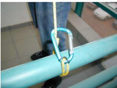
The line can be attached to large objects such as building pillars/columns by passing the line around the pillar and clipping it back onto itself.
